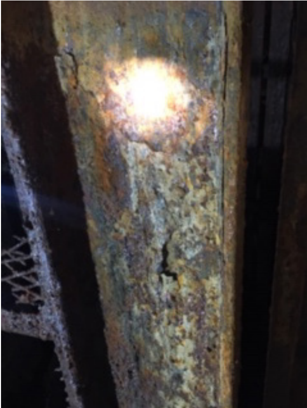
Figure 1: Steel before being cleaned Source: Euroz
