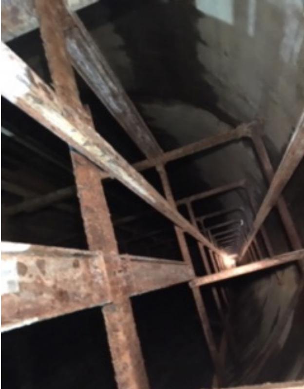
Figure 3: Looking down the 8.8m diameter shaft Source: Euroz
